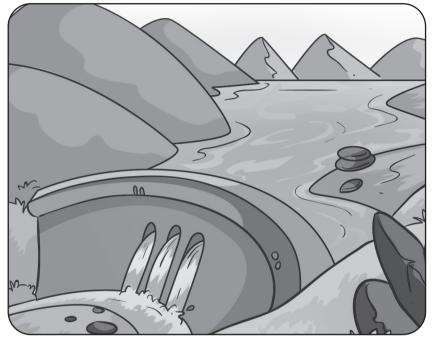
• The pressure acting on a dam at the bottom of a reservoir, for example, is greater than the pressure acting near the top. As a result, dam walls are typically wedge-shaped.
